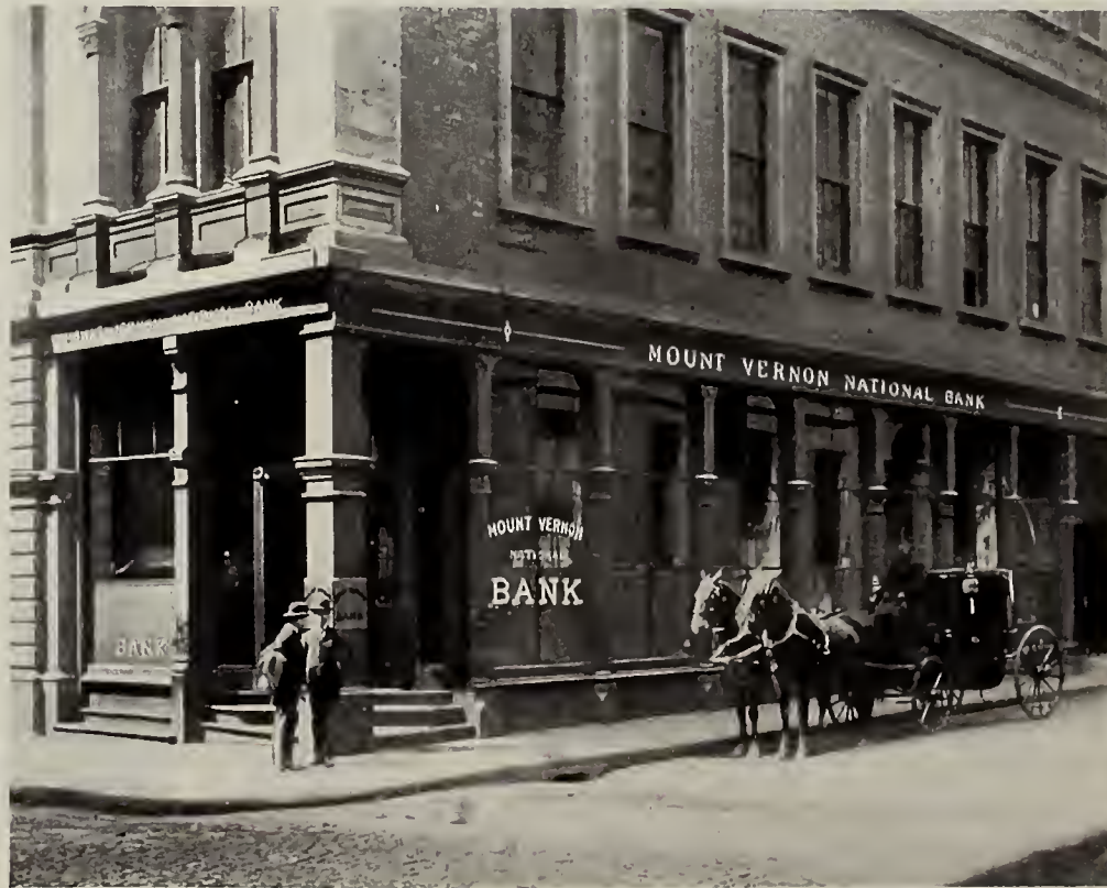
MOUNT VERNON NATIONAL BANK, 43 Chauncy Street.
